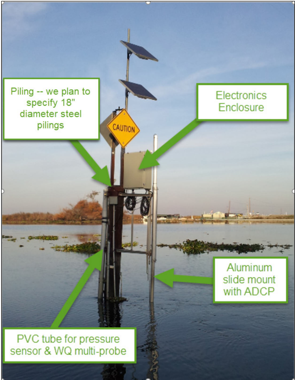
Figure 2. Standard Configuration of a Delta Flow and Water Quality Monitoring Station
